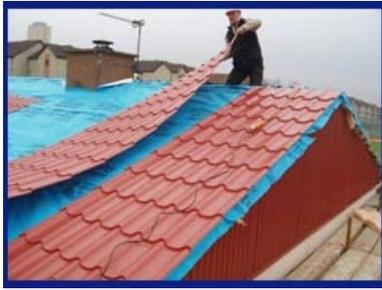
Position and fix Versasteel 1100 sheets from ridge to eaves, taking care to align the sheet square to the ridge / eaves axis and not parallel to the gable. To assist, an Alignment Board can be fixed at a distance of 40mm from the front face of the eaves fascia and the tile sheets fixed accordingly. Tile sheets to be fixed down to battens with Self Drill, Tap Fasteners minimum 25mm long with EPDM or Neoprene Sealing Washers or special Fixings for fixing to steel purlins.
